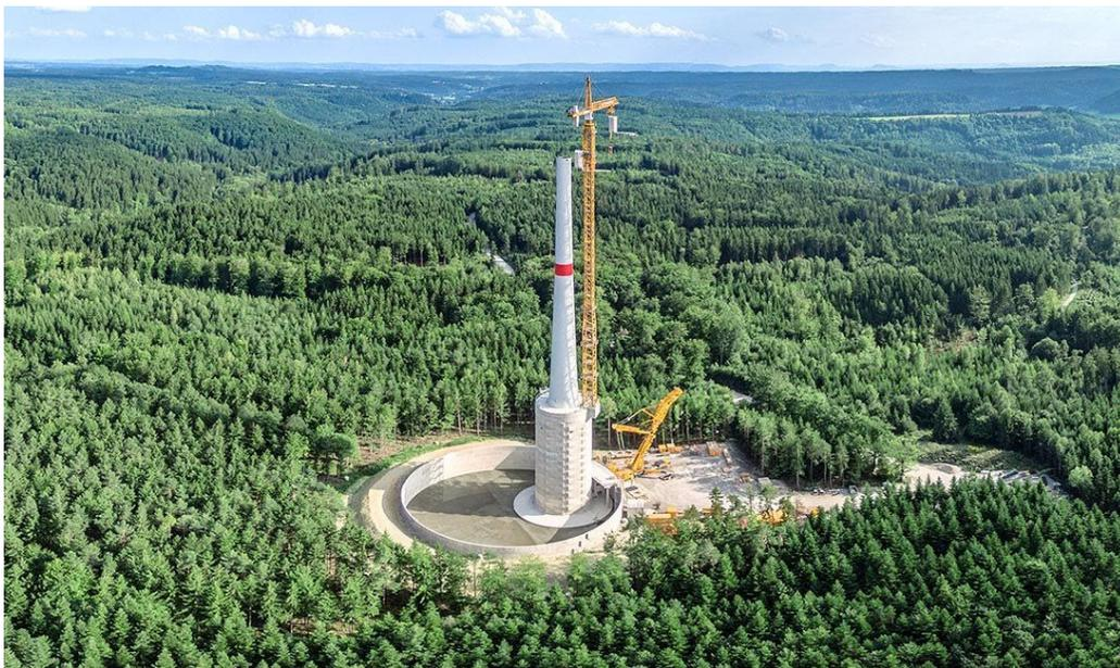
**Figure 3-7 Water Reservoir around the Foundation of Wind Tower (Source: Max Boegl website, <https://www.mbrenewables.com/en/pilot-project/>)**
