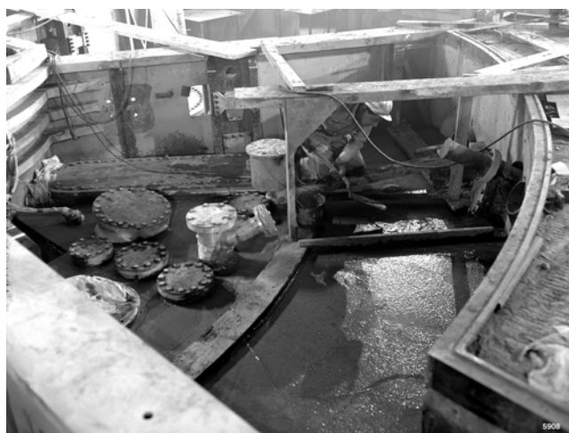
FIGURE C-22. CONCRETE AND THE UPPER SUPPORTING STRUCTURE.
