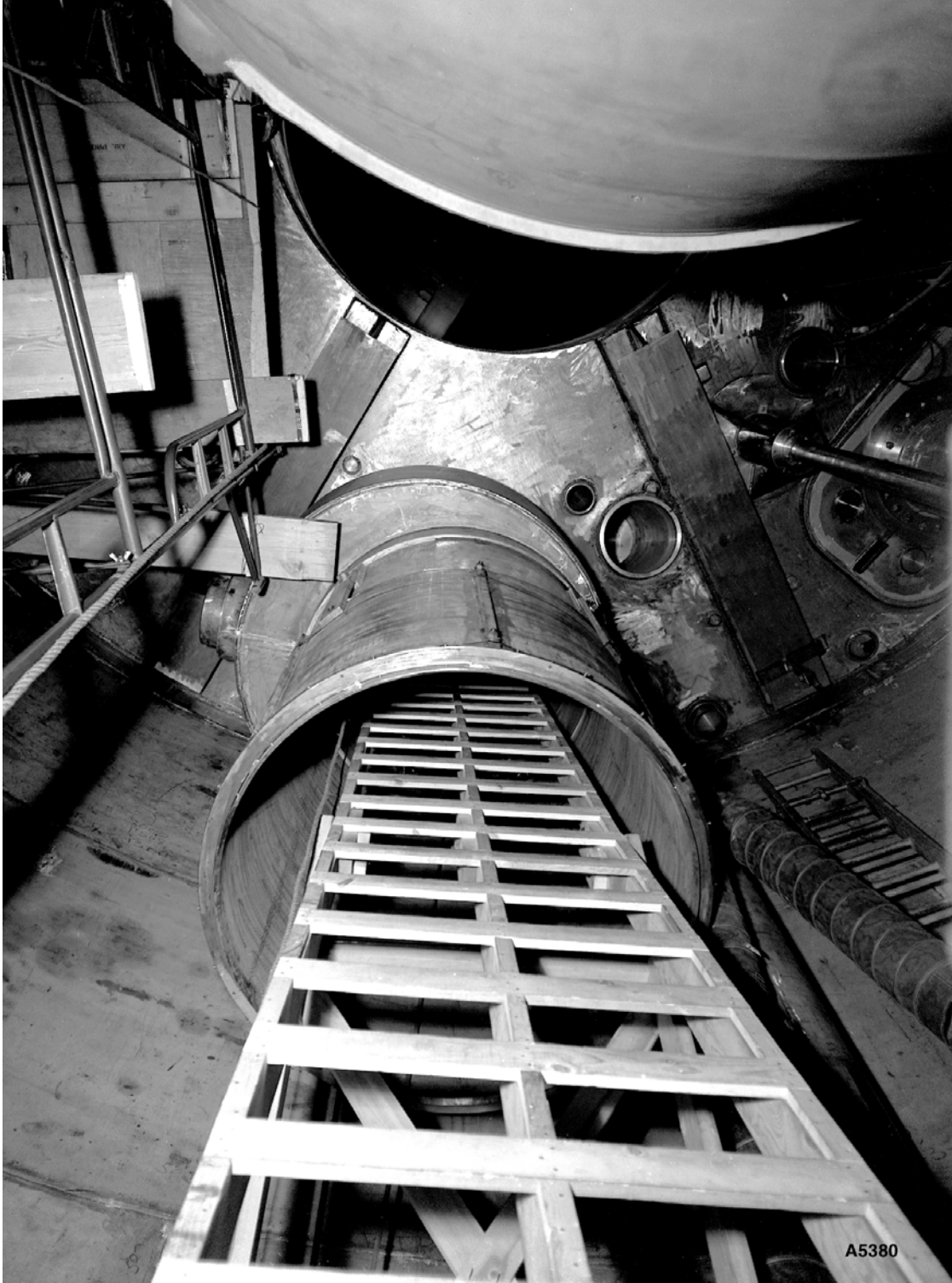
FIGURE 2-16. OPEN NOZZLE FOR THE IHX (LOOKING UP).
