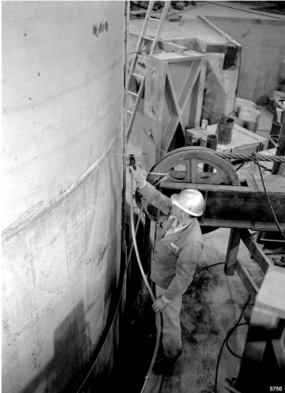
FIGURE C-11. INNER TANK WELDS BEING LEAK TESTED.
