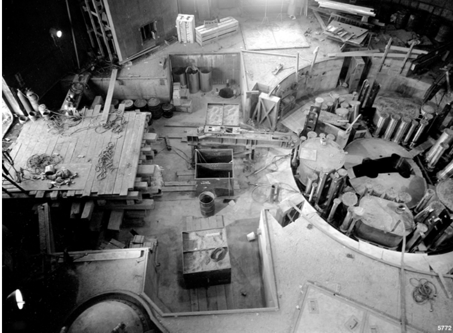
FIGURE C-15. PRIMARY TANK IN POSITION IN THE BIOLOGICAL SHIELD CAVITY.
