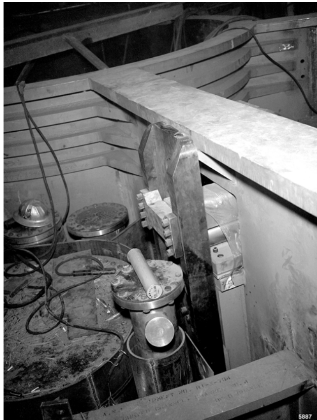
FIGURE C-19. PRIMARY TANK PRIOR TO CLOSING THE UPPER STRUCTURE.
