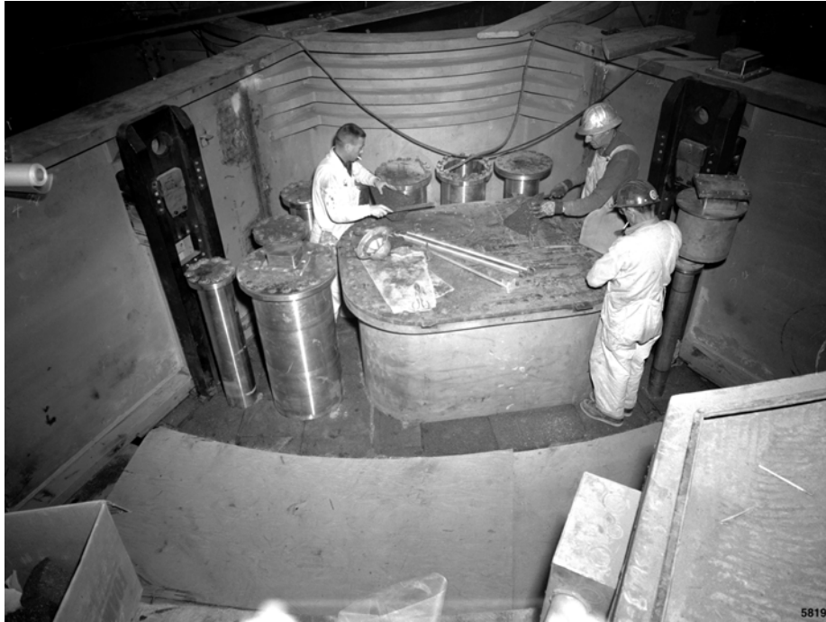
FIGURE C-19. PRIMARY TANK PRIOR TO CLOSING THE UPPER STRUCTURE.
