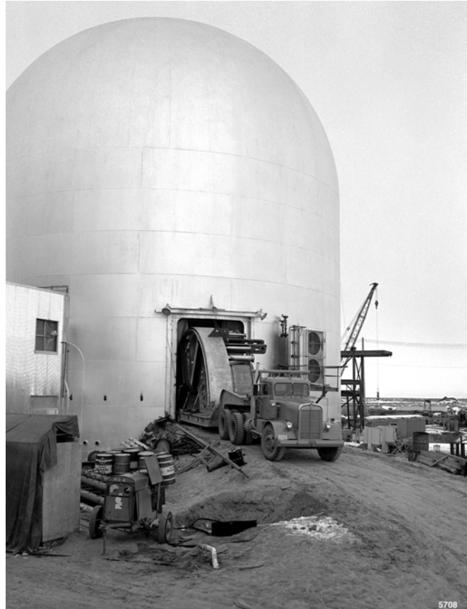
FIGURE C-4. ONE HALF OF THE PRIMARY TANK COVER ARRIVING AT THE EBR-II SITE.
