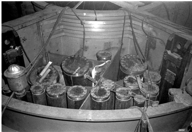
FIGURE C-21. SLEEVES IN THE PRIMARY TANK.
