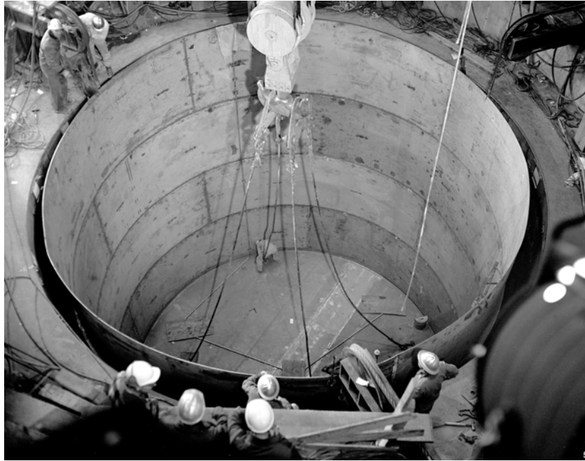
FIGURE C-6. OUTER SAFETY TANK POSITIONED IN THE CAVITY.
