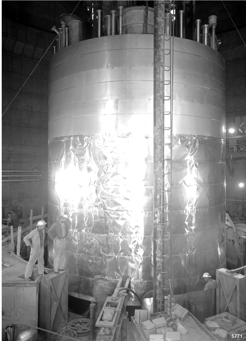
FIGURE C-14. INSTALLATION OF THE INSULATION NEARLY COMPLETED.
