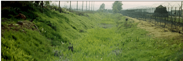
Example of a typical drainage ditch
