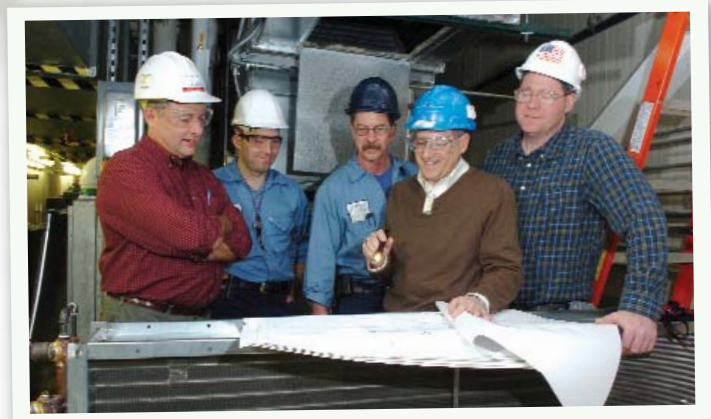
Top: Example of storage ring air-temperature fluctuations before (red) and after (blue) air conditioning upgrades. Bottom photo: AES and FMS personnel conducting an in-progress review of construction activities in preparation for commissioning of the upgraded storage ring air conditioning system. Left to right: Rick Janik (AES), Robert Brachle (FMS), Glenn Willes (FMS), Marvin Kirshenbaum (AES), and Andrew Stevens (AES).
