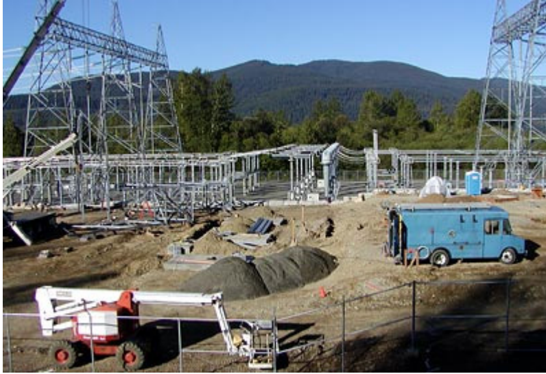
FIGURE 1.7-9 Substation under Construction (Source: BPA)
