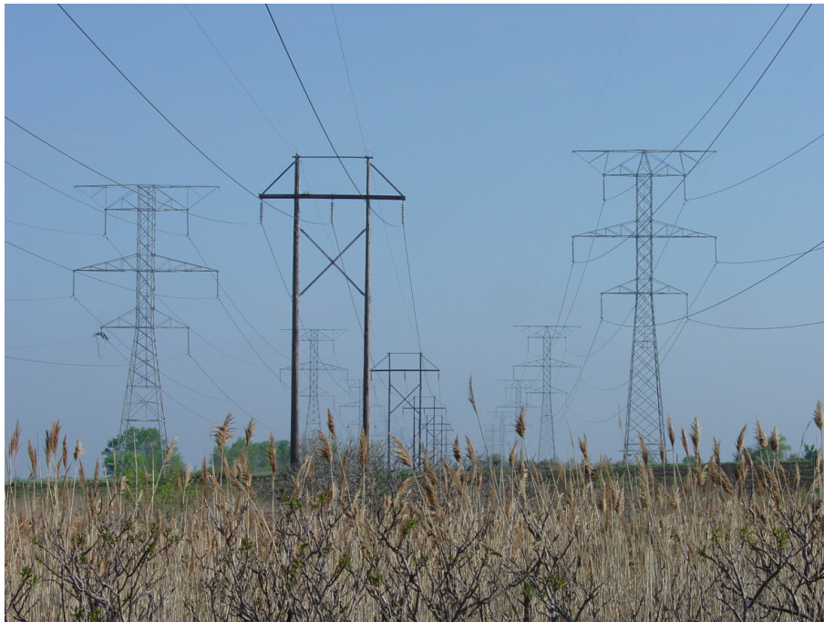
FIGURE 1.6-2 Multiple Lines in a Power Corridor (Source: Argonne Staff Photo)
