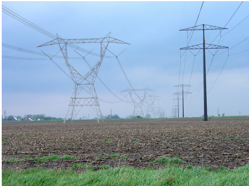
FIGURE 1.6-1 Lattice (left) and Monopole (right) Towers (Source: Argonne Staff Photo)
