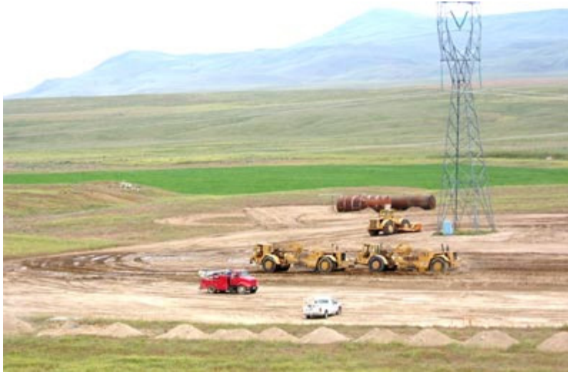
FIGURE 1.7-2 Site Preparation for Construction of Substation (Source: BPA)
