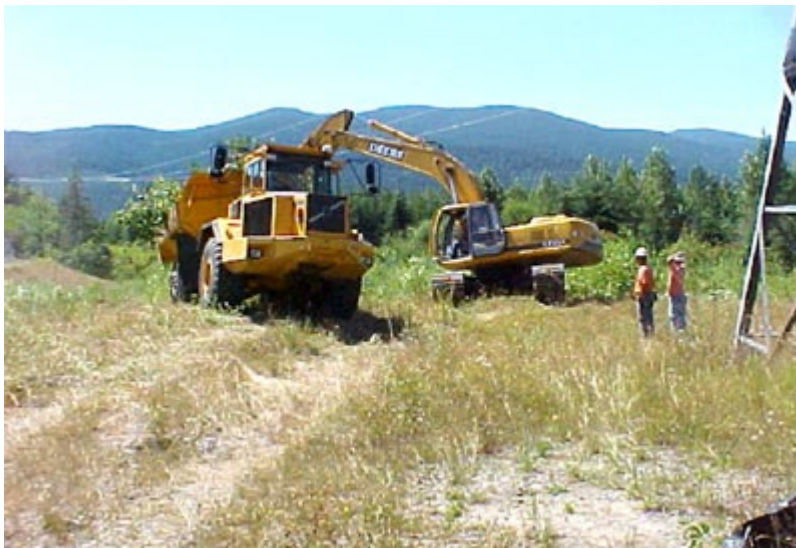
FIGURE 1.7-1 Clearing Vegetation for Expansion of Kangley-Echo Lake Substation (Source: BPA)
