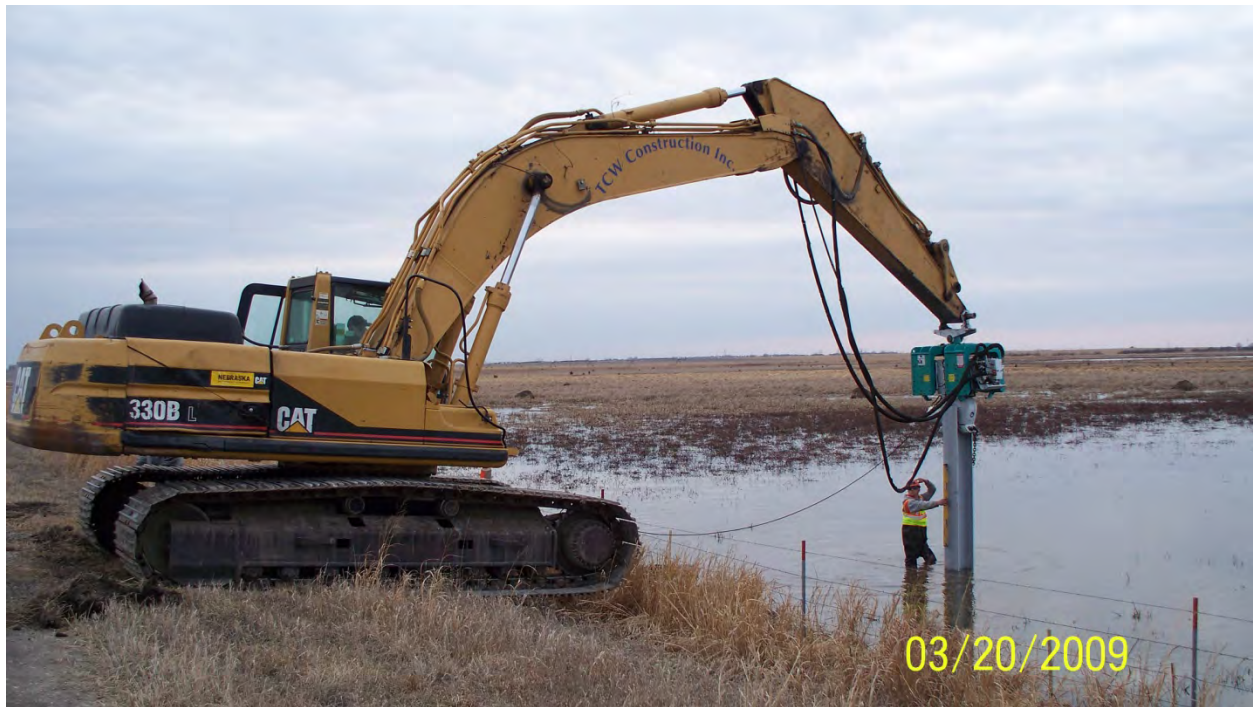
FIGURE 6.2 Installation of H-piling in the north wetlands subbasin to support a permanent water level gauging staff, March 2009.
