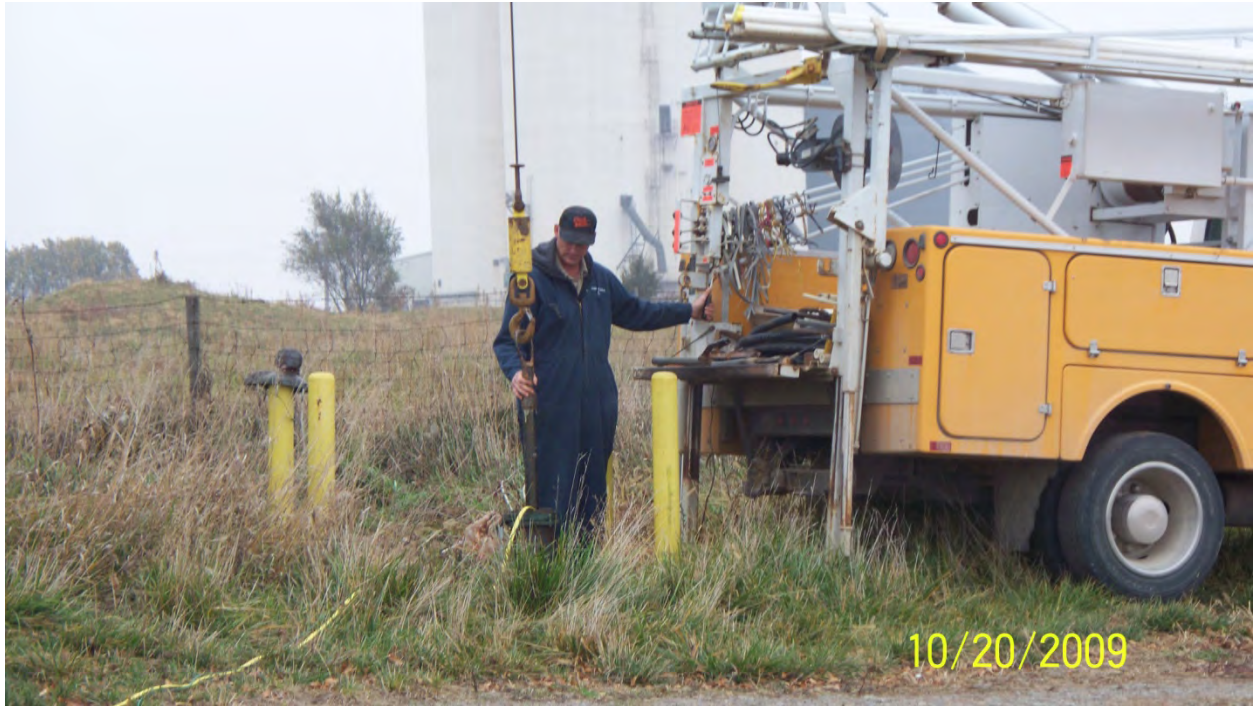
FIGURE 3.1a Servicing of extraction well GWEX4, October 2009, by personnel of Webster Drilling, Inc.
