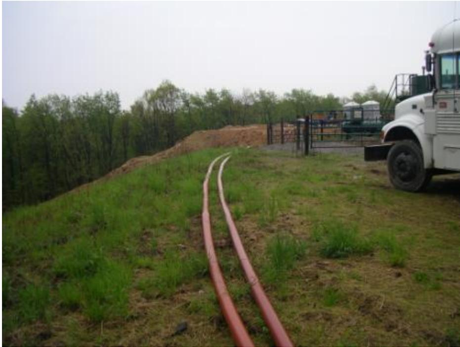
**Figure 14 – Aluminum Pipe Used to Convey Water**
