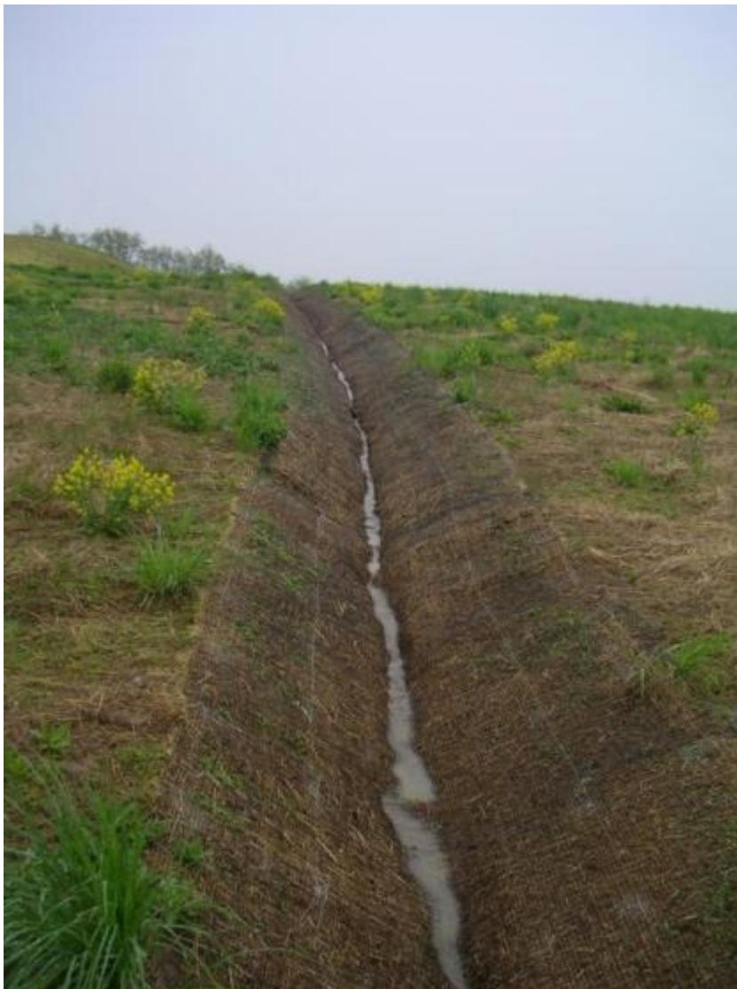
**Figure 9 – Lower End of Stormwater Diversion Ditch**
