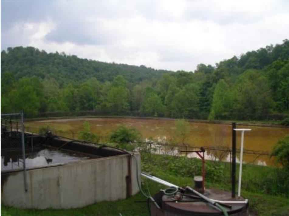
**Figure 31 – Aeration Tank – with and without Anti-Foaming Chemical – Tunnelton Liquids**
