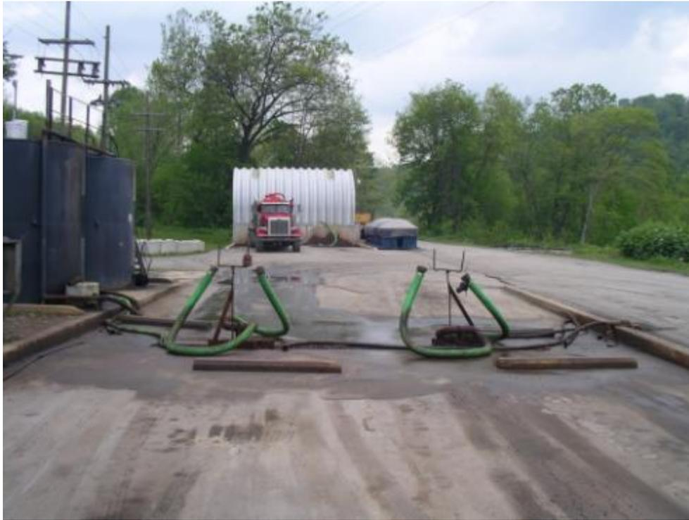
**Figure 29 – Oil/Water Separator – Tunnelton Liquids**
