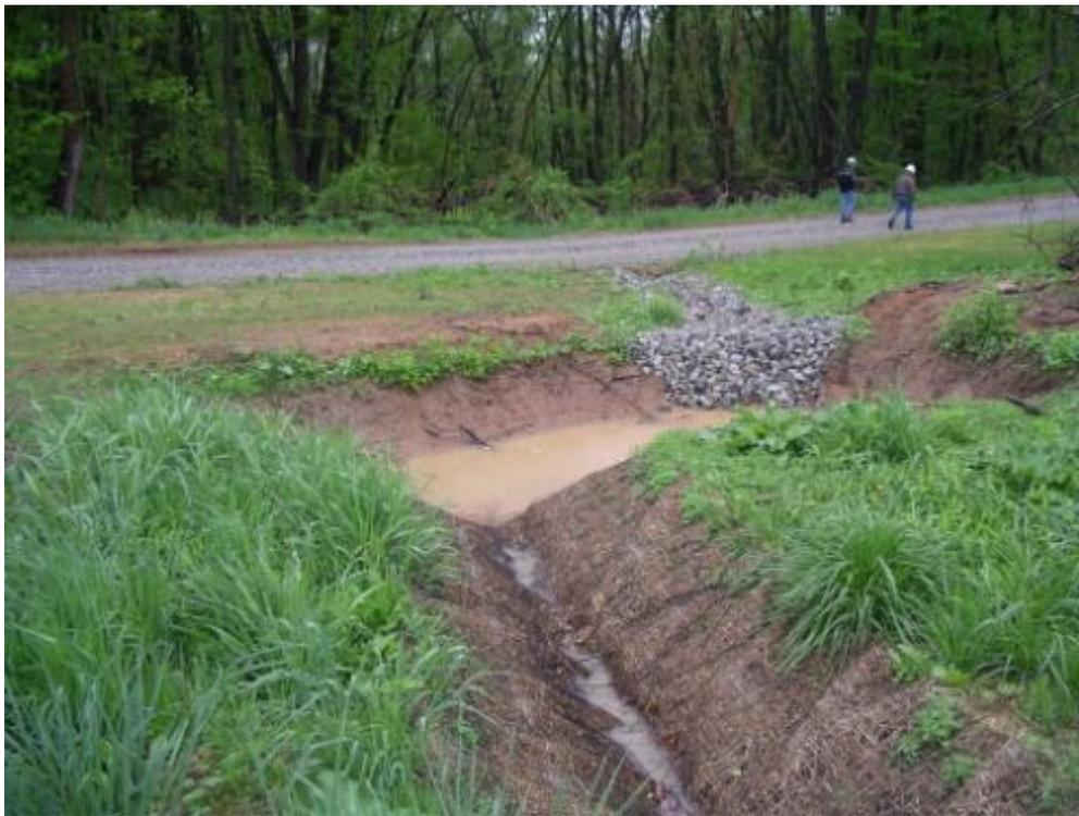
**Figure 10 – Stormwater Control Structure**
