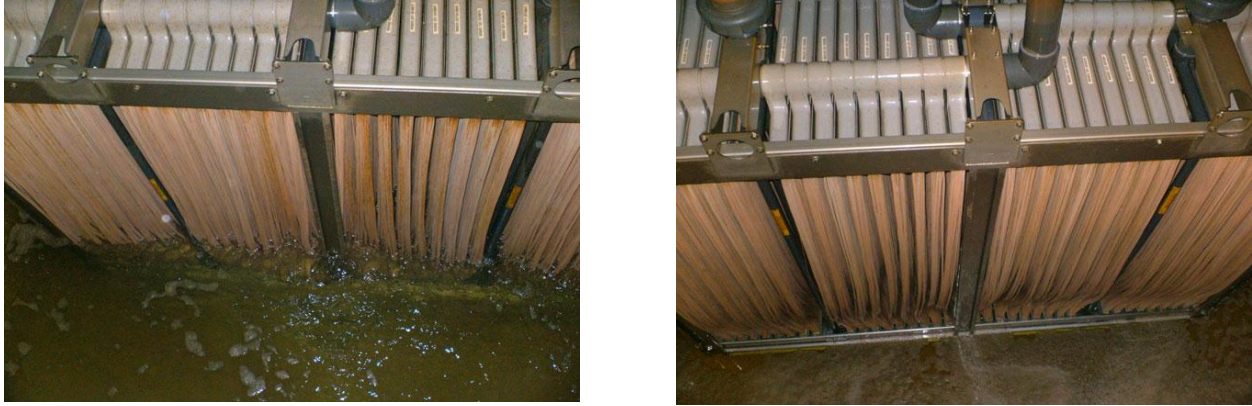
Figure 2.8 Membrane Cassette Before and After Recovery Cleaning (Bergman et al., 2006)[6]
