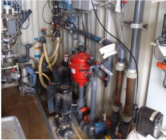
Figure 3.3 Wastewater Feed Pumps (left) and Chemical Feed System (right) (Permission to use photograph granted by Blue Water Technologies Inc.)
