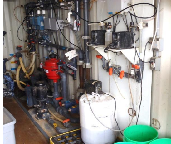
Figure 3.3 Wastewater Feed Pumps (left) and Chemical Feed System (right) (Permission to use photograph granted by Blue Water Technologies Inc.)
