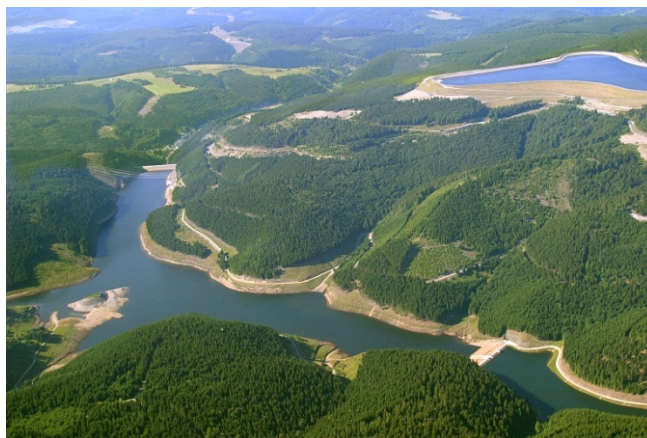
Figure 2-2 Goldisthal Pumped Storage Project in Germany (Source: Vattenfall GmbH)
