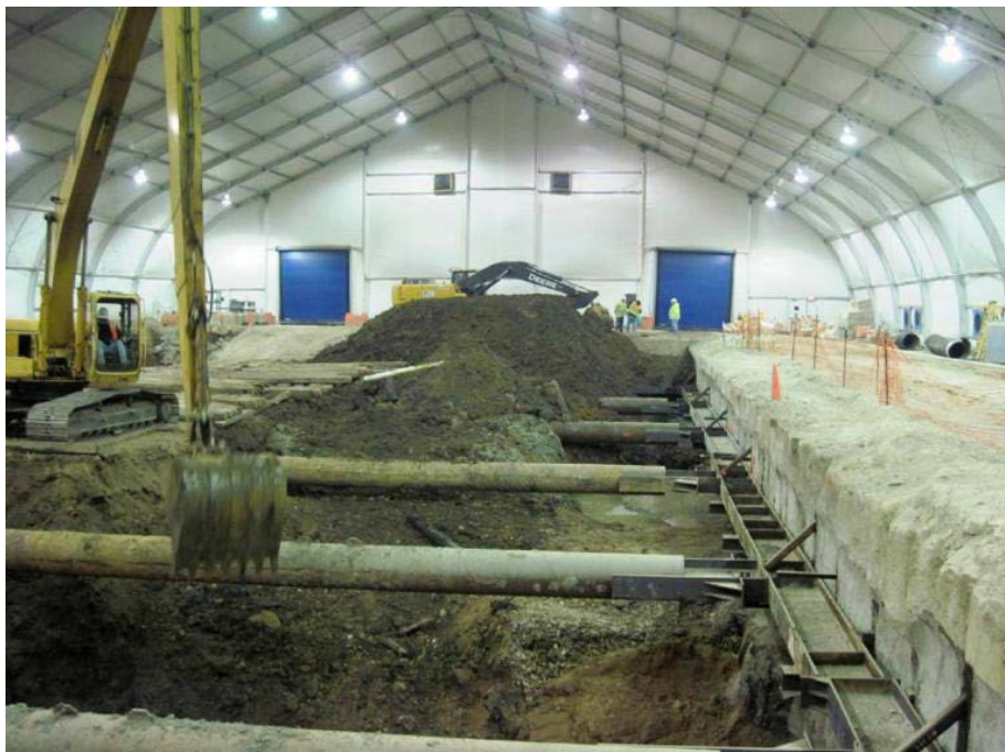
FIGURE 5-11 Example of Containment Structure (Source: Mahaffey Fabric Structures 2015)
