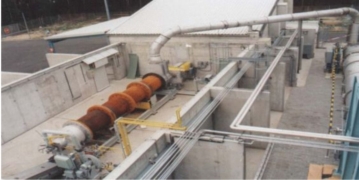
FIGURE 5-10 Sprewerk Lubben (ISL) Rotary Kiln Incinerator (Source: Wilkinson and Watt, 2006)
