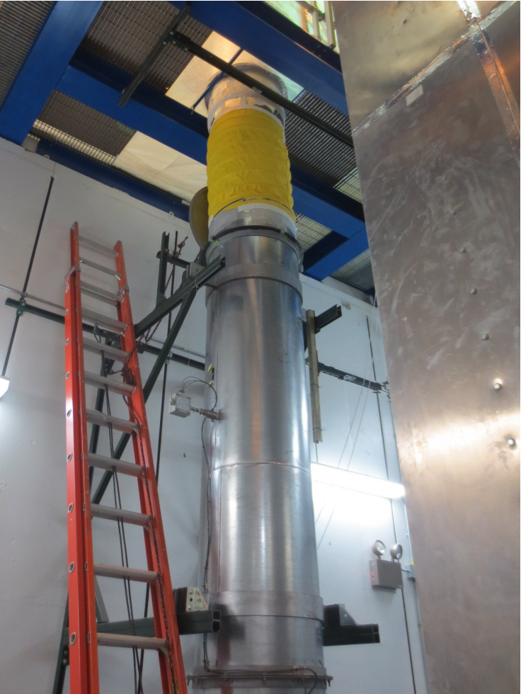
Figure 102: Extension from argon enclosure to inlet
