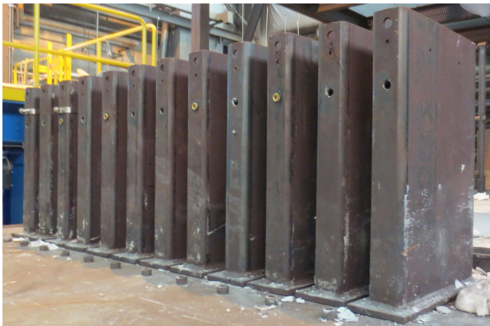
Figure 122: Exposed riser ducts (outlet) after removal of upper plenum, August 2016
