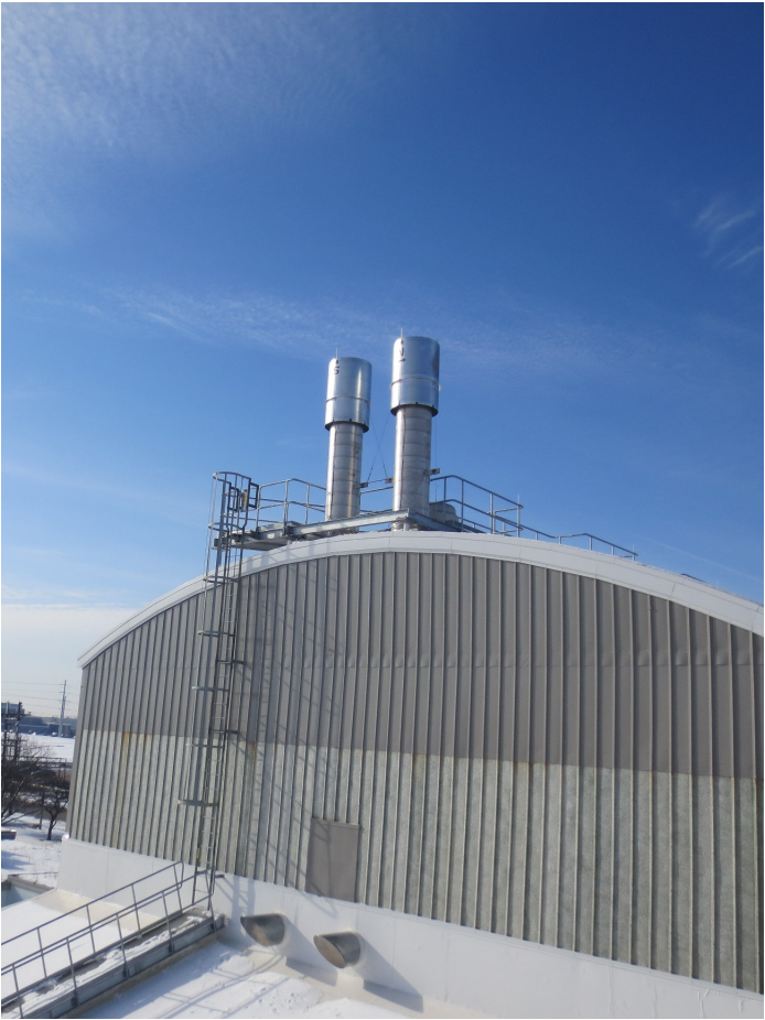
Figure 117: New caps installed, Bldg. 308
