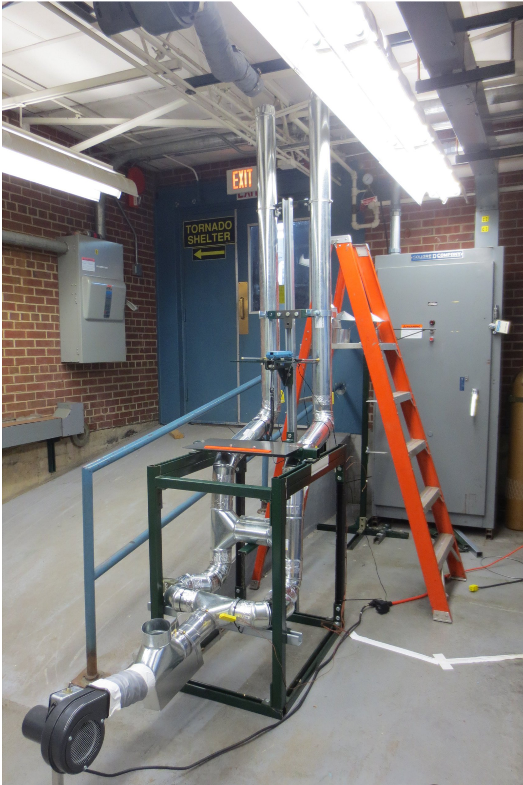
Figure 114: Picture of 1/12, chimney duct-work only, forced flow mini-NSTF
