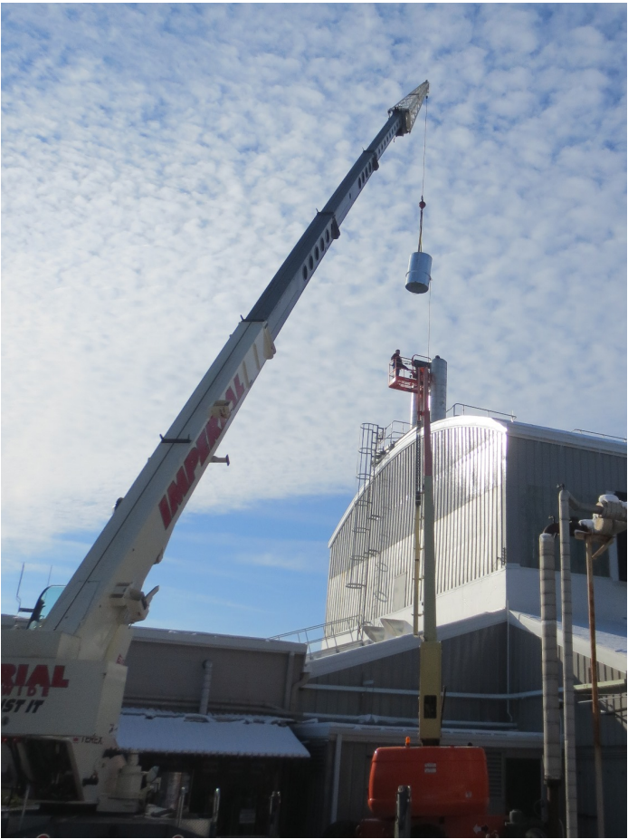
Figure 116: Installation of new caps
