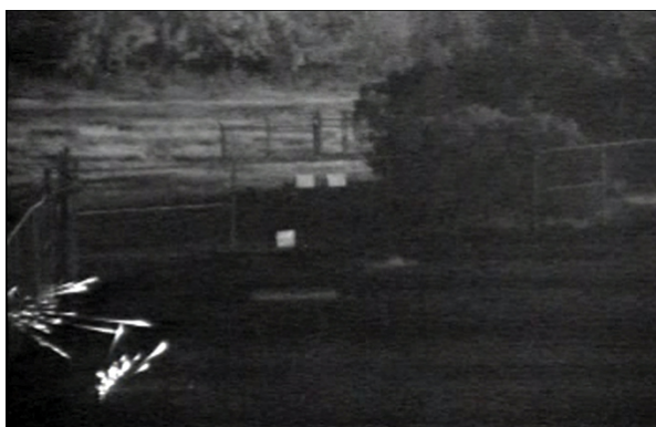
Figure 5: Gunfire Attack Captured on Metcalf Substation Security Camera 24
