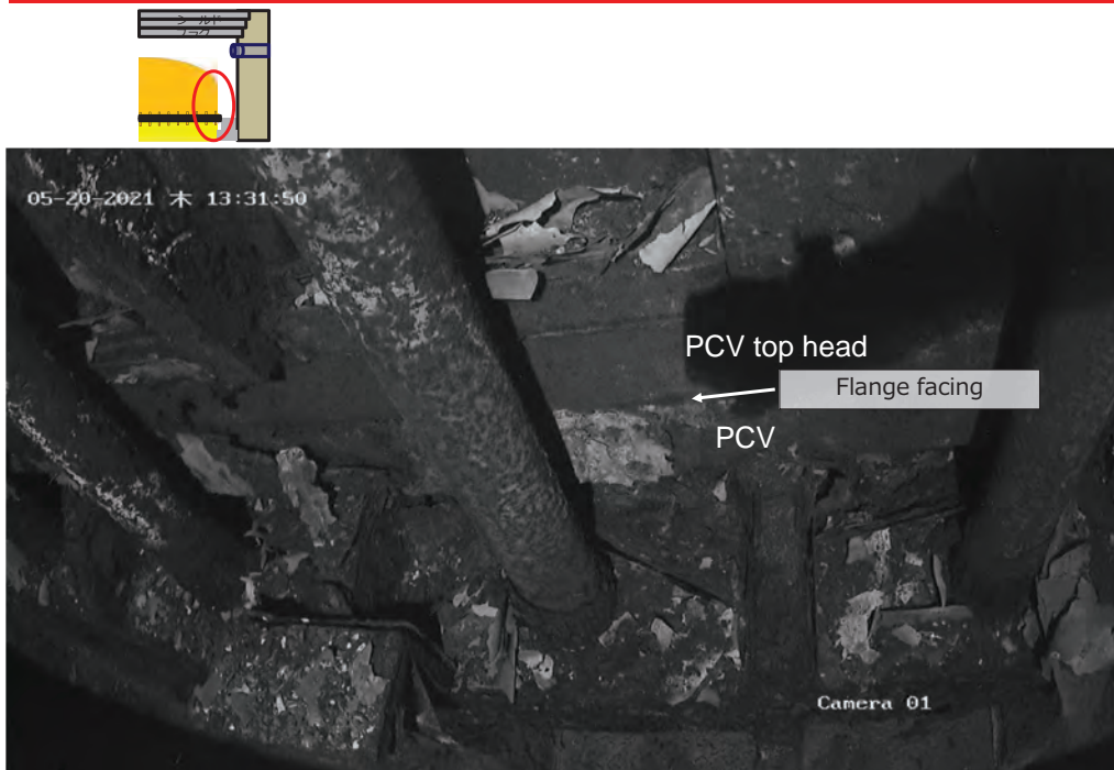
(Picture) PCV flange joint
