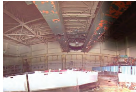
Paint extremely deteriorated at 2011/10/20
