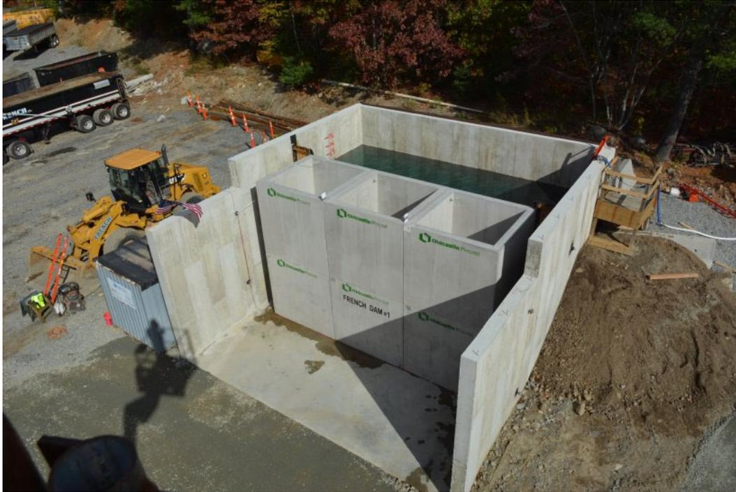
**Figure 5-7 Precast Modular Dam Prototype (Source: DOE)**
