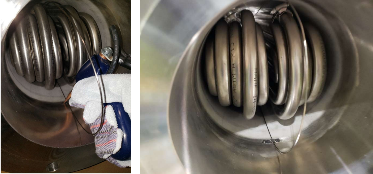
Figure 36: Photograph showing the installation of fiber capillary tube installation on shell side of AHX
