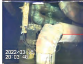
RCW piping near PCV penetration (under water)
