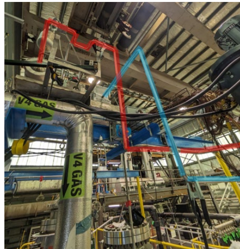
Figure 3: Photographs showing the THETA secondary system components installed on the platform structure (left) and the hot return and cold supply secondary sodium piping (right). Note the hot return and cold supply sodium pipes have been highlighted with red and blue, respectively.
