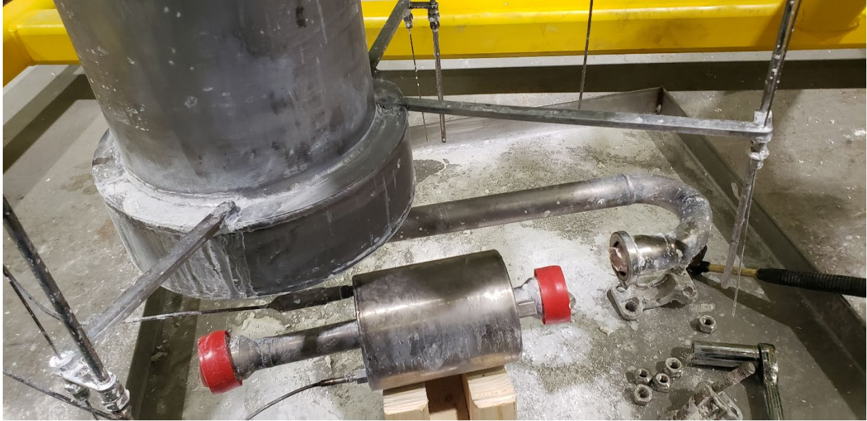
Figure 31: 1" Grayloc connections removed from either side of flowmeter.
