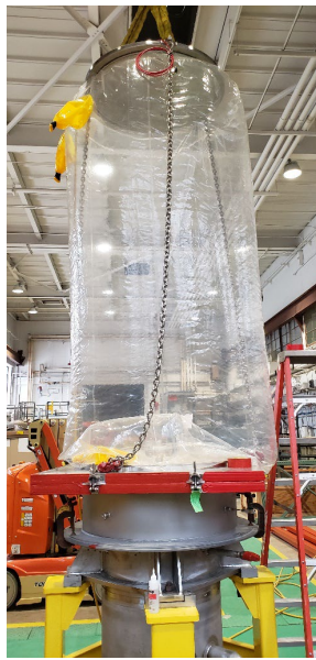
Figure 16: 28” Flexicask being tested with air to ensure glovebag and gate valve assembly gaskets are all working correctly
