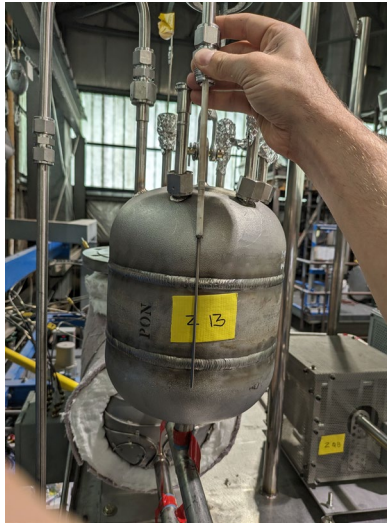
Figure 68: Expansion tank without trace heat or insulation showing the relative position of the lower conductivity probe level sensor.
