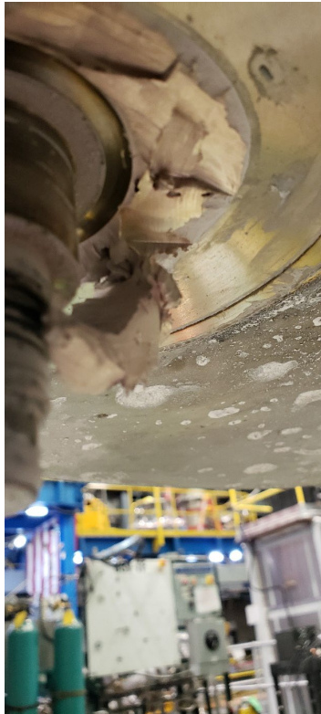
Figure 30: Labyrinth seal with pump shaft protruding, left. Labyrinth bottom plate removed and sodium scraped from the bottom of the vessel, middle. Sodium being cleaned from the shaft to allow for top portion of labyrinth seal to be removed, right.
