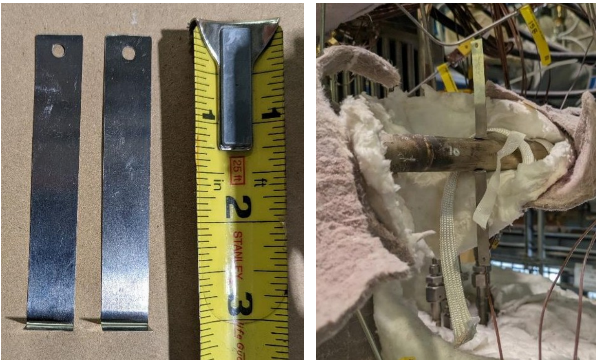
Figure 10: Photo showing voltage measurement leads made with 316ss sheet metal, left. The leads as installed on THETA secondary system are shown in the right photo.
